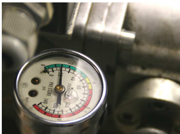
Gauge showing the pressure during filtration process (image 3)
